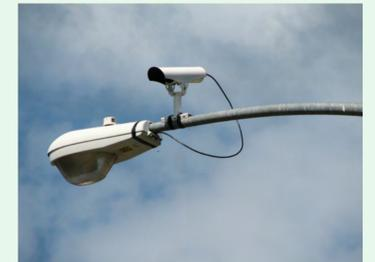
At many signalized intersections, cameras detect vehicles and bicycles and trigger the green light.
